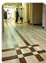
A combination of Stratica's Antique Rosewood and Elm seen here at the Fresno Surgery Center in Fresno, Calif. The manufacturer notes that this resilient flooring is non-PVC and chlorine free, as well as eco-polymeric. The company notes that it is well suited for a health care facility.
