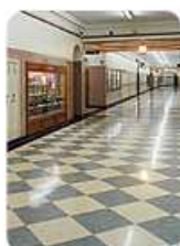
Forbo Marmoleum Tile installed at a high school (Photo by Beth Singer Photography).
