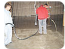
Poured underlayment can be a big time saver over multiple coats of troweled patching compound. Photo courtesy of Pyramid Floors
