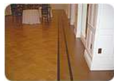
A beautiful herringbone cork tile installation done with contact adhesive.
