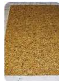
Fiber reinforced underlayment with cork installed over it.
