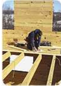
A plywood subfloor is installed directly over the floor joists and is part of the structure of the building. Photo from www.quiltbus.com .
