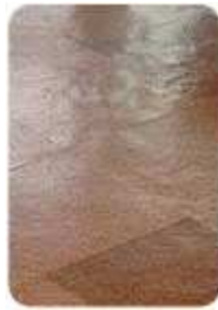
Proper substrate preparation will prevent telegraphing of substrate irregularities.
