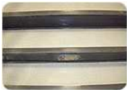
Stair nosings are installed much like stair treads and have added strength if epoxy is used at the nose. In this installation, 1/8" VCT is used with rubber stair nosings and risers.
