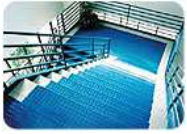
This is a nice use of two colors of stair tread material and rubber tile on the landing. This photo also shows one way of seaming a stair tread with the seams placed out of the traffic area. Photo courtesy of Roppe.
