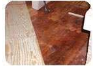
A/C Plywood being installed over an unsuitable plywood subfloor. (Photo courtesy of Mickey Moore - FCI October 2004)
