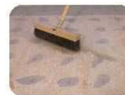
It may or may not be necessary to patch the joints and fasteners on the underlayment - check with the manufacturer to be sure. (Photo courtesy of Tarkett)
