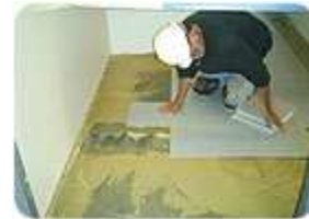
Although relatively easy to install, the difference between a good VCT job and a not-so-good one is usually time. (Photo courtesy of Pyramid Floor Covering)
