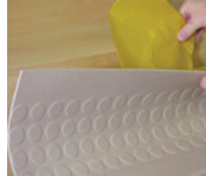
Photo 4: Then, gently fold the tread back and remove the release paper from the back of the tread.
