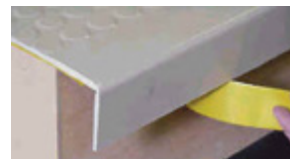
Photo 3: When using the tape system, first remove the release paper from the nose of the step and set the tread against the step edge.
