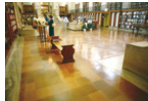
This installation mixed several colors of natural cork tile in a random pattern.
