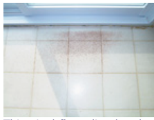
This vinyl floor discolored because of exposure to direct sunlight. (Photo courtesy of Tarkett's Jef Silfies and John Coppola.)
